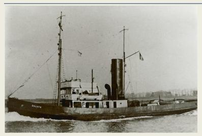
Belgian commercial tug operating under Dutch ensign. Allocated to SNO Portland to tow Bombardons. Built 1921 by SA des Forges & Chantiers de la Méditerranée, Le Havre. L131.3'. B28.6'. D13.9'. 3cyl 340grt. 1200ihp TE 14.5"x23.5"x36.5"x27"s engine by builder. Callsign OLKV later OTGA later ORMC later MGRA. 2-1922 Delivered to French Government, named L'etalon. 1925 Sold to SA de Remorquage à Hélice,
