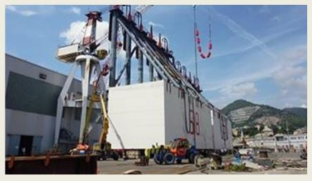
Work in progress at Giglio complete installation of S5, the eight of the 15 sponsons to positioned starboard side of the Concordia. In the meantime, remediation activity on sponson S13 have been completed in Genoa and the sponson is ready to depart from Genoa on board pontoon
