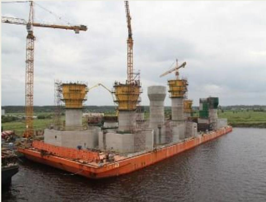
The humble flat-top barge in all its permutations is a much neglected vessel type (yes, at DSB we do indeed consider a barge to be a 'vessel!') and yet they are the workhorses of the industry. Largely non-propelled, unglamorous and often uncomplicated in design, nevertheless, the flat-top barge is an essential piece of marine equipment on many marine construction projects worldwide. Jan De Nul's 'DN143', however, stands out from the crowd as a
