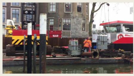
vessels. The pontoon was then brought up with injected air. The slanted crane, which was half on it, was very slowly driven completely ontp the deck of the work ship. It was now hoped that the work on the Korte Engelenburger Quay could be resumed at the end of this week. (Source: Vesseltracker; Photo: RTV Rijnmond))
