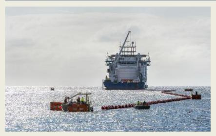
An export cable for the 600MW Kriegers Flak offshore wind farm made a successful landfall at Rødvig, Denmark, Energinet reports. The cable pull-in operations were carried out with NKT's cable laying vessel - NKT Victoria. Energinet constructing onshore and offshore infrastructure connect Vattenfall's Kriegers Flak wind farm in the Baltic Sea to the Danish grid. The
