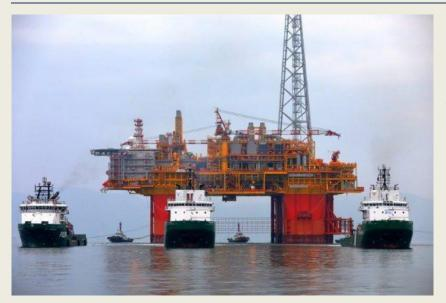
Japan's Inpex has informed that the central processing platform for the Ichthys gas field has arrived in the Australian waters of the Browse Basin today. The massive Ichthys Explorer platform weighing 120,000 tonnes and with topsides measuring 130 meters by 120 meters, is considered the world's largest semisubmersible platform. The Ichthys Explorer reached its final offshore destination,
