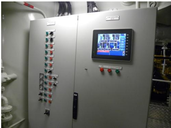
Electric power distribution board
