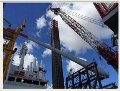
well in advance of its original schedule, the vessel now completed the installation of the first turbine. MPI was responsible for the design, engineering and manufacturing of the sea fastenings which will be used during the transportation and installation of all the above mentioned turbines. MPI also has and will continue to provide project management throughout the whole turbine
