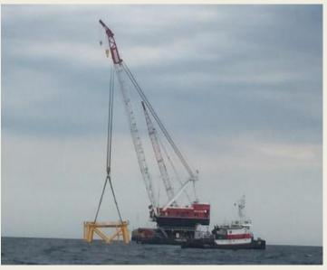
bad weather or repairs such as this one." The first jacket foundation was installed on Saturday by the floating barge crane, **Weeks 533**, while the whole foundation installation is expected to take eight weeks. After it is completed, the wind farm will produce enough clean electricity to power 17,000 homes. *(Source: Offshore Wind; Photo: Jeff Grybowski/twitter)*
