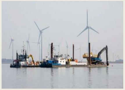
wind farm. "In total, we have installed 48 inter array cables between the wind turbines and six export cables that connect the offshore wind farm to the mainland," said **VBMS** spokesperson. the Now, the company is doing the terminations, connecting the cable to the turbine, which should be completed early August. Nico Verburg, project manager VBMS said: "Despite the exceptionally bad weather during the cable installation period,
