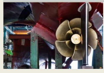
The 26 meter, all aluminum, catamaran version of the Fast Crew Supplier is called the **FCS 2610** "Twin Axe." The below vessel has been designed to best enable workers to transit to, and board offshore wind farms for maintenance. The image shows two that are currently being constructed. Edwin de Smets, Yard Manager at Damen Shipywards Singapore notes each FCS 2610 takes approximately 34 weeks to build from start to finish. *(Source: gCaptain)*
