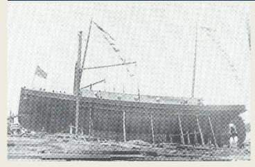
The **Charles W. Parker Jr.**, rigged for Lunching in 1909 at Bath, Maine. She was much the same as the Grenough: 125 feet long, 27 feet beam, 16 feet depth, 700 horsepower. Note the strapping holding her rudder for and aft, and the shores wedged against her lower rubrail. Just before the launch, the shores are knocked away. There is a bunting-draped platform at her bow, with a temporary set of stairs leading to her stem. The stairs are for the convenience of the
