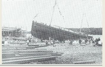
stern quarter. This is an active shipyard. In the background is another vessel, most likely a schooner, in frame, and in the foreground are a number of timbers for the next building project. All the debris on the ground is wood chips left from many years of wooden shipbuilding. In some yards, the accumulated chips formed piles several feet deep. *(Source: On the Hawser by Steven Lang and Peter H. Spectre)*
