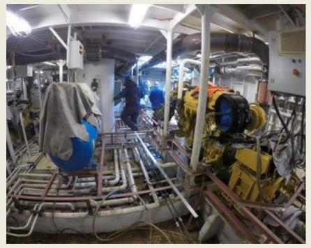
Since the arrival of the hull of our newest vessel Shoalbuster Barney, a lot has been done. The last 6 weeks the shipyard worked hard to ensure they would make the delivery date of 1st of May 2015. And all the hard work they put in is showing, especially in the engine room and the accommodation. Both air have compressors been installed as well the sewage plant. In the aft peak the installation rudder is already in place and some of the floor plates are in place.
