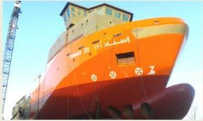
The sections of our yard number 470 are assembled, over 70 meter of hull is standing on the slipway, the engines and thruster units are placed and so are the electric switchboards and many other key components and pieces of equipment. This means that the first vessel of a series of 10 PSV's is taking shape. Build activities are in full swing and every day more workers join on board. With the
