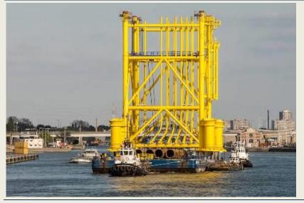
The Jacket for the substation Butendiek Offshore Wind Farm on was seen on the 18<sup>th</sup> April on it's way to be installed by Scaldis Salvage & Marine Contractors NV heavy lift vessel Rambiz. *(Picture taken by author: Alan Cuypers)*
