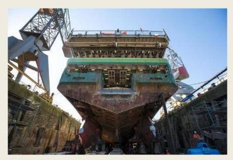
the ship are supposed to last about 35 days, according to Flip van der Waal, General Manager Shipdock Amsterdam. The work scope consists of Ballast Treatment Water installation, installation of a new workboat and davits, relocation of the MOB and a 5-year special survey. Polarcus Naila, a vessel which combines the latest developments in maritime systems with the most advanced seismic
