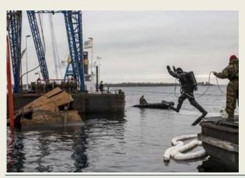
specialists are dividing the wreck into 3 segments. This is being done with explosives and hydraulic tools. First they had to remove a metre of sand and clay from the vessel, which was equipped for laying mines. Then the military hydraulic engineers could cut the deck in half and break away the first segment. They then made cuts in the segment for the hoisting beams, with which the wreck segment was brought to the surface. (*Press Release*)
