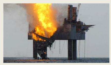
had recently been preparing the well for production when natural gas came flowing out of the well. The natural gas caught fire short time later а developing into a large blaze. The Hercules 265 suffered significant damage as the fire caused part of the rig to collapse. The beams supporting the derrick and drilling rig floor have fallen
